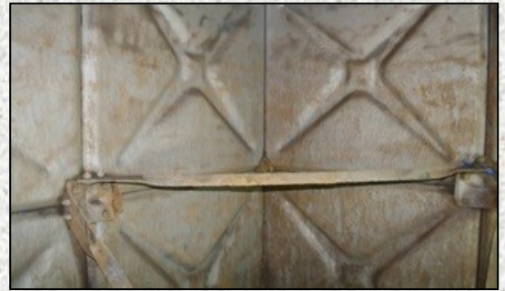
After Surface Preparation
