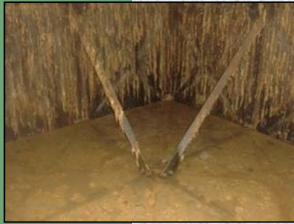
Before Surface Preparation
